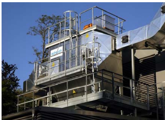
Electrostatic precipitator of a biomass heating system with a heat power of 2 MW (fonte wikipedia)
